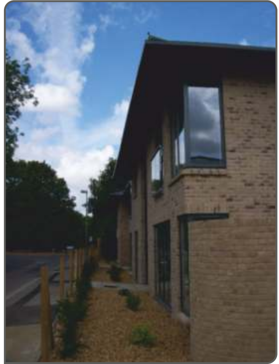
Architectural detailing (Station Road, Ramsey)
