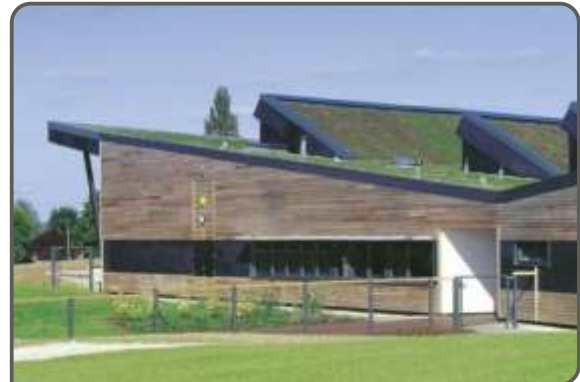
Primary school, Great Notley, Essex (CABE) Designed through a design competition and uses a sedum roof and modern methods of construction
