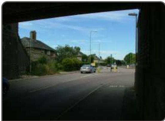
1. View to Cambridge Road through railway bridge
