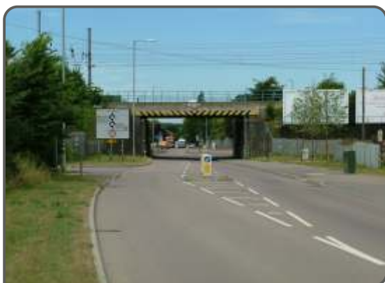
2. View to the railway bridge from Cambridge Road
