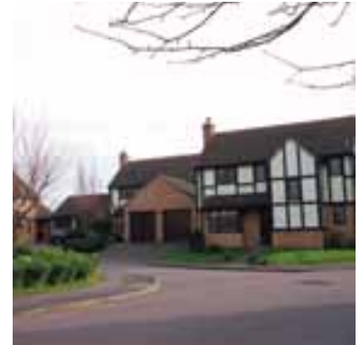
Housing at Crowhill is typical of recent development to the south of Godmanchester.
