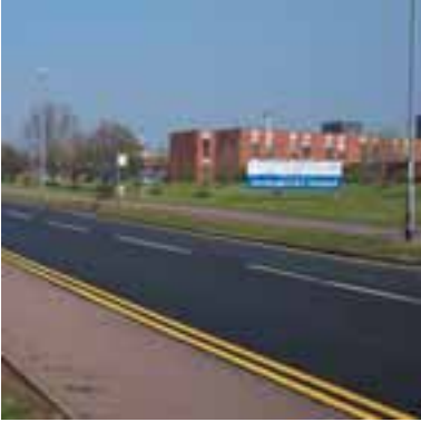
Hinchingsbrooke Hospital dominates the character of the main spine road.
