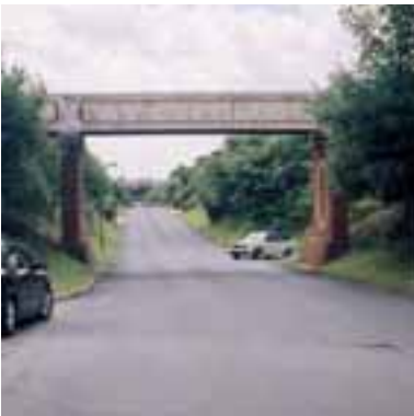
Visually intrusive footbridges across Coneygear Road.
