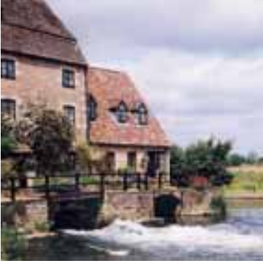
Water Mill at Water Newton. Note the use of limestone for wall and roof construction.
