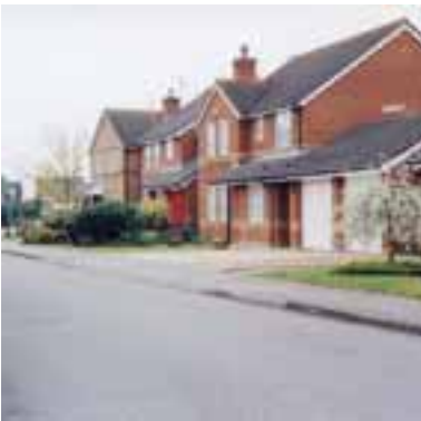
Recent housing to the north of Ramsey is typical of much recent development.
