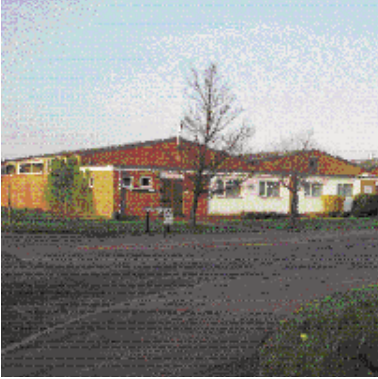
The older industrial estates are dominated by roads and large scale buildings.
