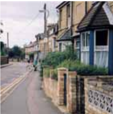
A mix of short terraces and semi's overlook the cemetery on Priory Road.
