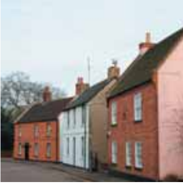
Earning Street: historic buildings create a strong sense of place and a village character.
