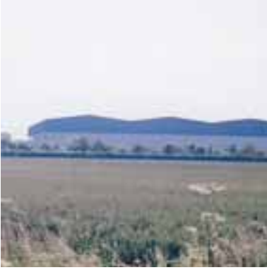
Large-scale buildings alongside the A1 at Alconbury Weston are very intrusive in the landscape.
