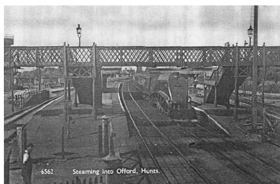
Buckden and Offord station. The platforms and pedestrian bridge have been removed from the site following the closure of the station in 1959.
