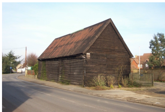
Barn at Fitz Farm - Weatherboarded with iron roof
