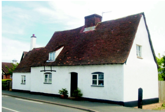
207 High Street - Timber-frame, rendered and tiled (The introduction of modern tile to the roof of Inglenook cottage is detrimental to the distinct character of local roofing)
