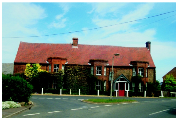
Whitwell Farm -18th century with 19th century alterations - red brick and red peg tiles
