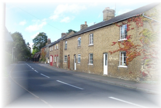
19th century cottages about the path to the street on the approach into Offord Cluny from Offord Darcy.
