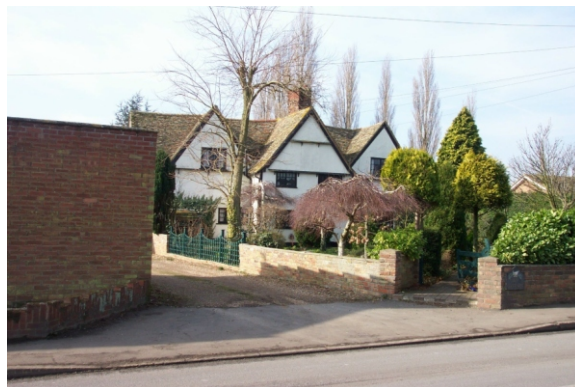
Ivy Cottage - timber-frame, rendered, peg-tiled.
