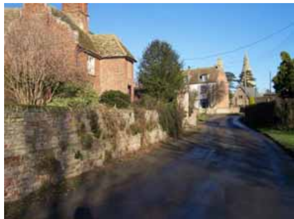
An impressive boundary wall at Bridge Farm.
