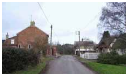
An otherwise attractive view into the Conservation Area disrupted by telegraph poles and overhead wiring
