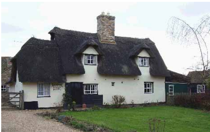
Right is a good example of a property that has retained a traditional window style and materials
