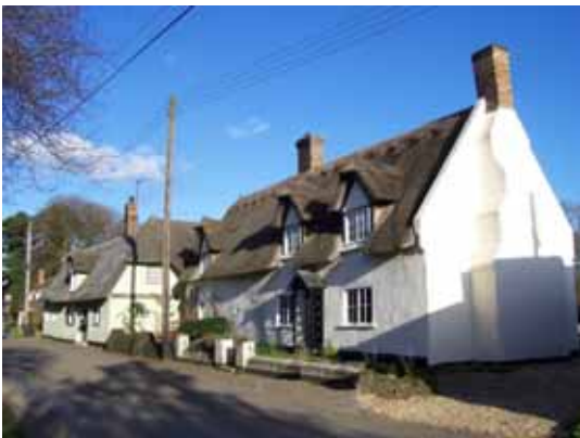
Brick Barn Cottage, opposite Birds Farm, is a typical example of the predominant architectural style in Broughton.
