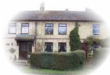
Modern alterations have had a detrimental effect upon the historic character of Too Loos House.
