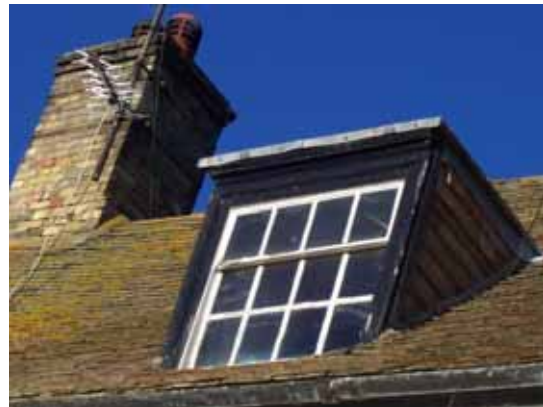
A flat roofed dormer at Birds Farm.
