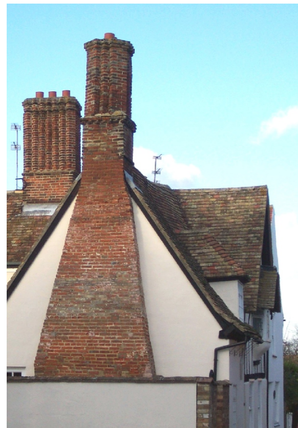
Chimneys at Plantagenet House
