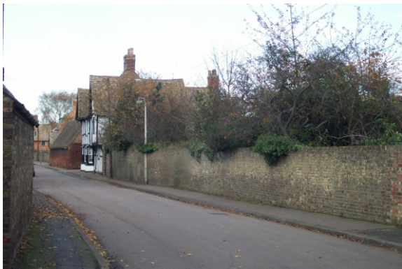
Boundary wall to The Gables
