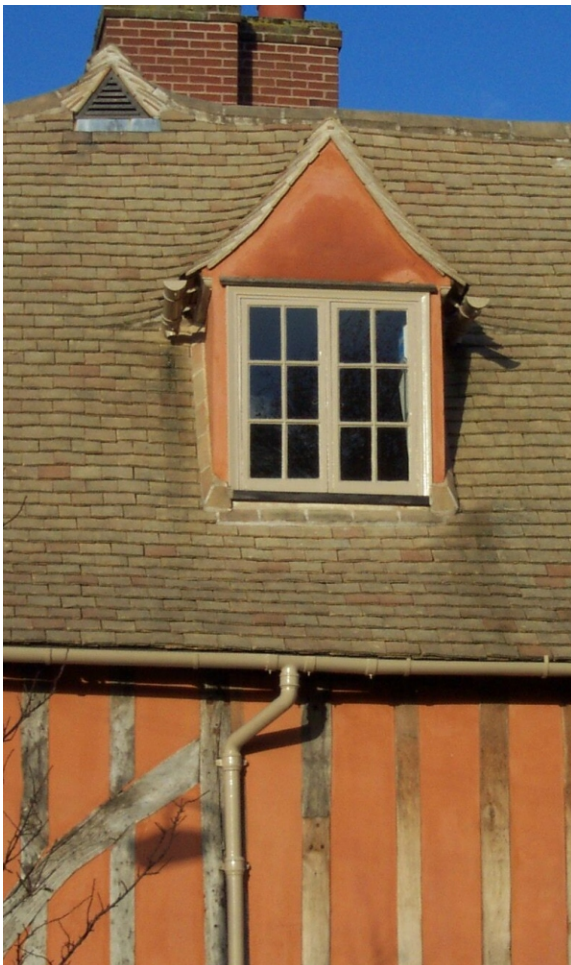
The timber frame, plain tile and gabled dormers of Tudor Farm
