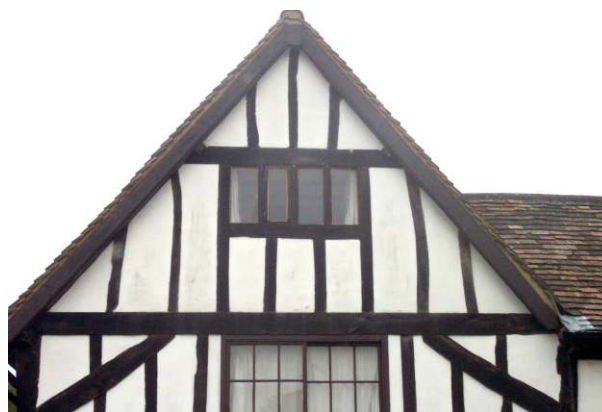
A timber mullion window in Old Court Hall
