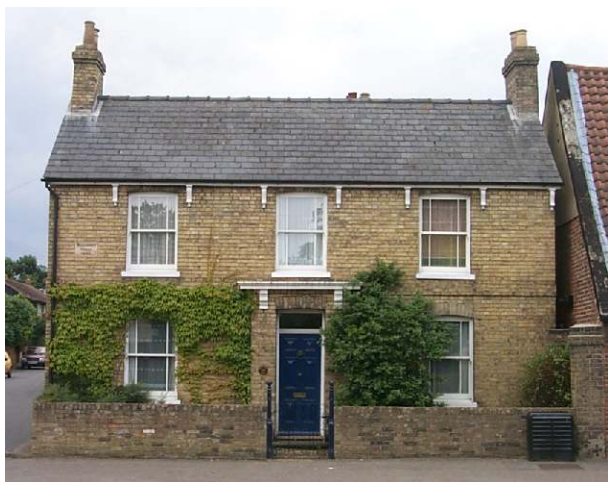
Victorian buff brick and slate - No. 31a Old Court Hall
