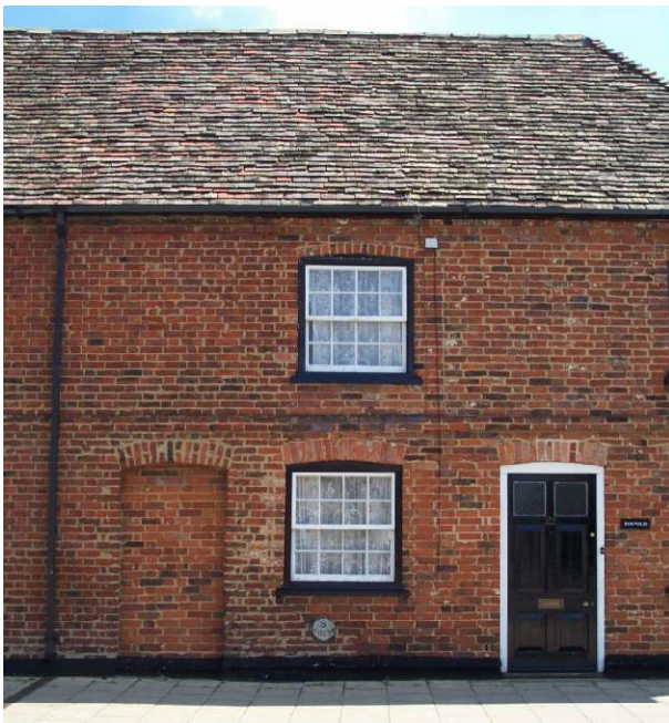
Georgian red brick & pegtile - Old Courthall.
