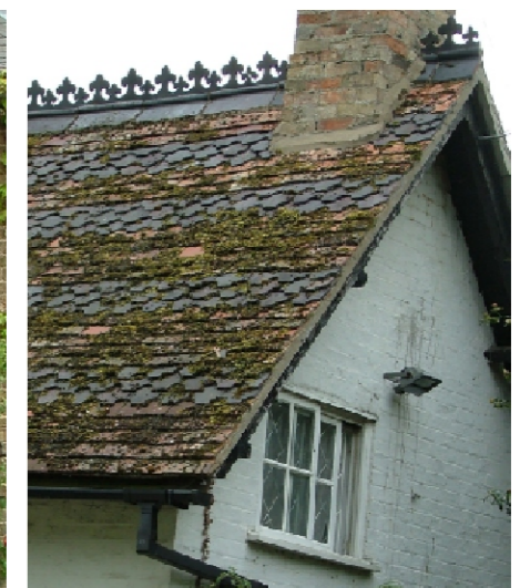
Later buildings were constructed of brick, sometimes painted. Clay roofing tiles were used on many later buildings, often replacing thatch on some older ones. Ridge tiles were a feature in many buildings.
