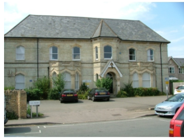
H. Priory House on the supposed sight of The Priory
