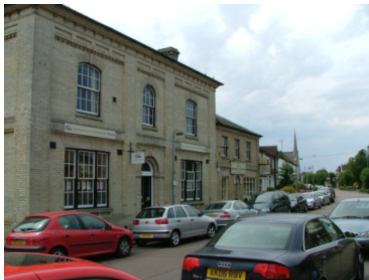
U. 19th century industrial and commercial buildings along Station Road
