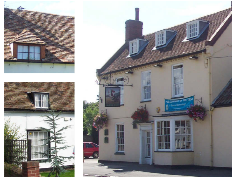
Vernacular cottages are found throughout the locality. Frequently rendered many will have internal timber frames. Clay-tiled roofs are typically punctuated with small dormer windows of varying design.
